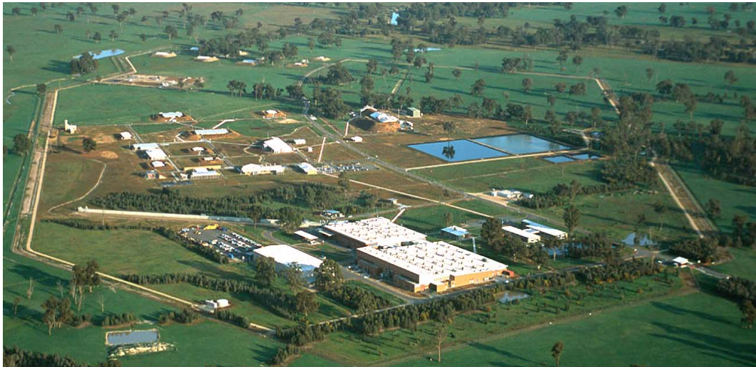
FIGURE 13. The Benalla site Circa 2003 set in rural surroundings north of the Benalla township. The main plant is in the foreground with magazines and other facilities in the background.
