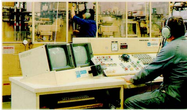
FIGURE 4. A View of the G+W plant from the operators console with the cartridge conveyor and tooling system behind the screens (from an AFF brochure)
